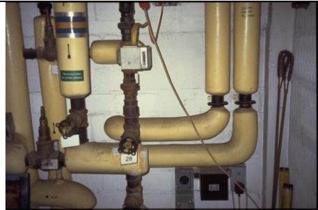
Moulded or preformed lagging - generally used in thermal insulation of pipes and boilers.
